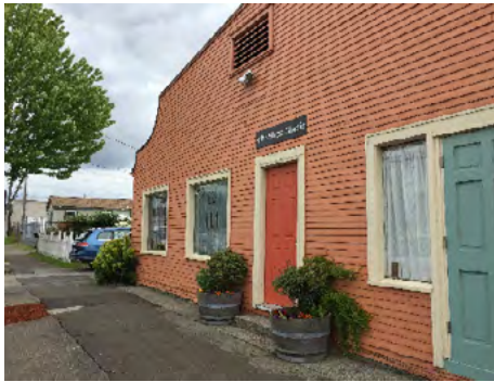
49th Street Studio, exterior
